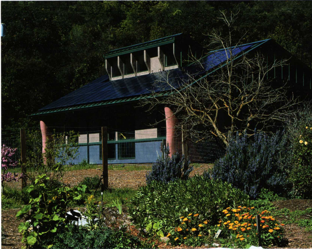
The roof of the southernmost wing of the building supports a photovoltaic system that produces as much electricity on an annual basis as the Wolken Center uses.
