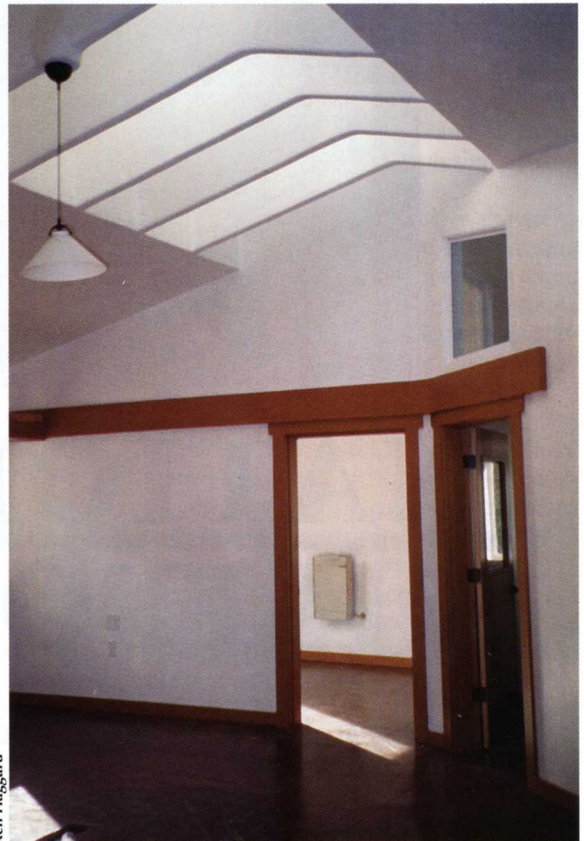
Continuing the prefabricated roof trusses through the dormer helps the system maintain its economic advantages and provides a series of finned lighted openings that distribute natural light without glare.
