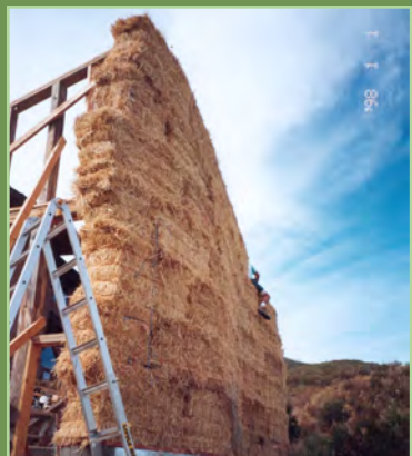
Utilizing straw bales to create fire resistant walls and expressive architectural form
